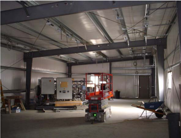
Figure 9. Inside look at the pilot plant building, October 2007.
