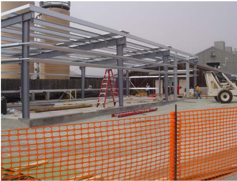
Figure 7. Framing the pilot plant building, August 2007.
