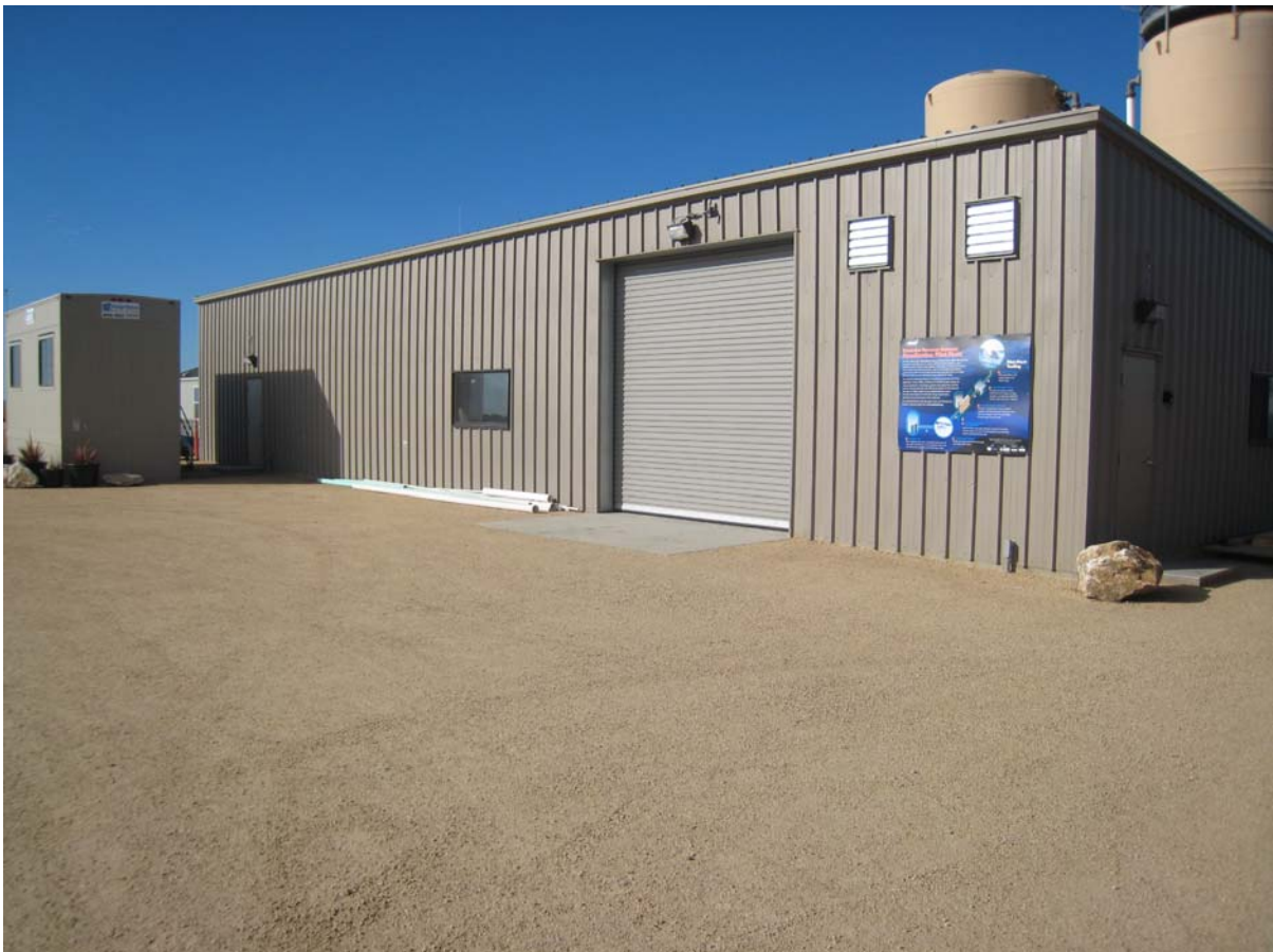
Figure 3. Seawater desalination pilot plant building located at UCSC Long Marine Laboratory, April 2008.
