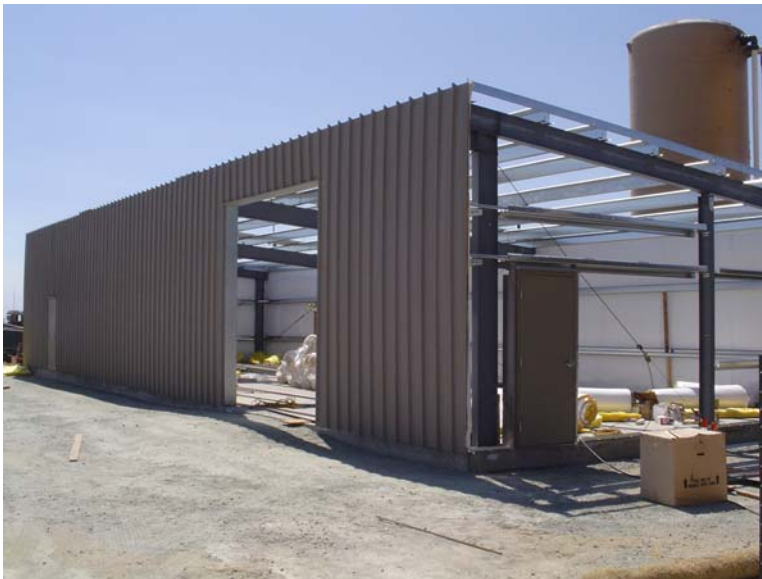
Figure 8. East wall of the pilot plant building, September 2007.
