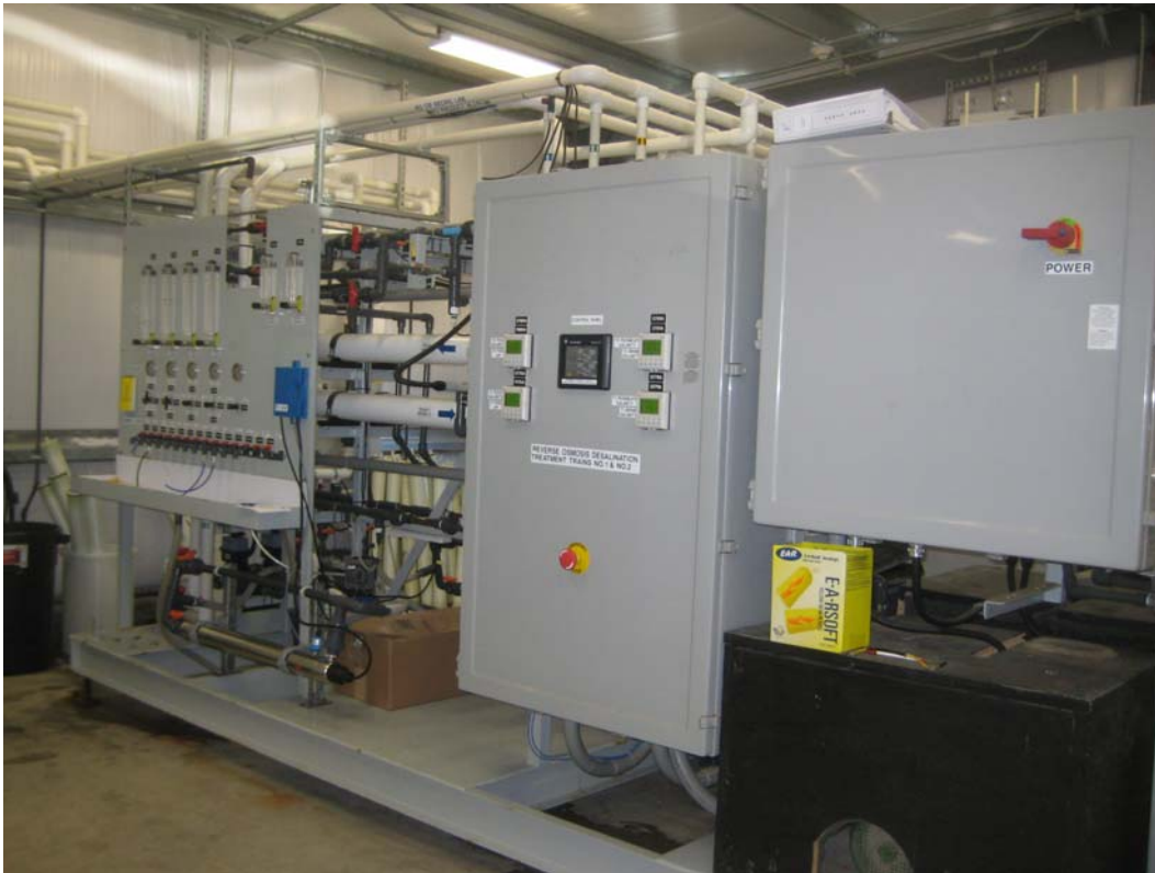
Figure 6. Monitoring panels used to collect data and compare the performance of reverse osmosis membranes.
