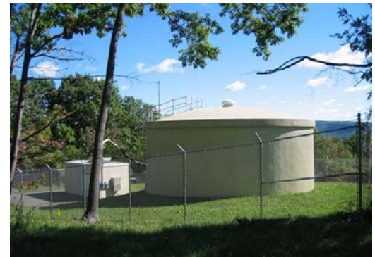
Above-grade concrete tank
