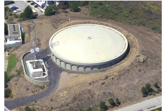
Partially buried concrete tank
