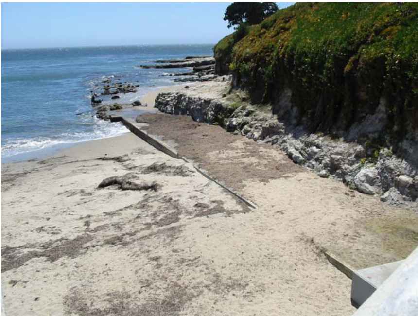
Figure 2-1. Offshore of Mitchell's Cove Beach is the location where a 0.6 km (2,000 ft) abandoned outfall pipe may be used for a screened, open ocean intake in sandy marine habitat.
