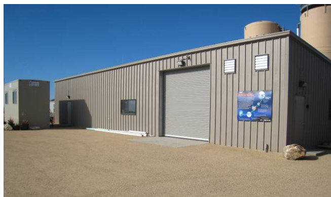
Pilot Plant Building at the LML
