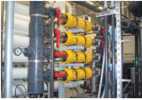
Innovative technology, such as energy recovery devices (above), reduce the amount of energy needed for the desalination process.
